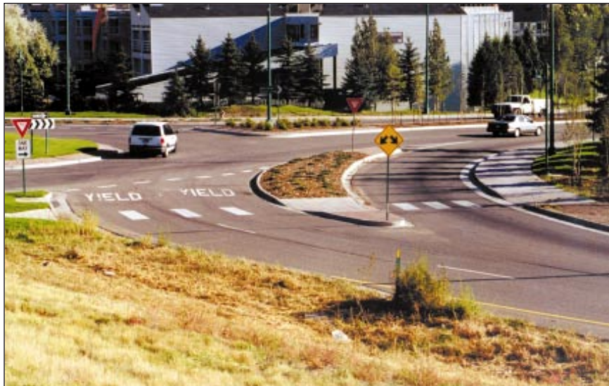
Exhibit 6-41. Example of right-turn bypass lane.
